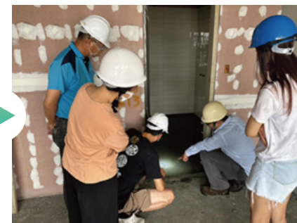
Waterproofing testing of each household's bathroom
