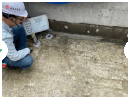
Roof slab waterproofing testing
